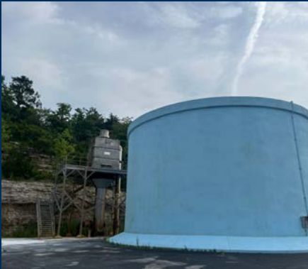
Additional finished water storage, to increase system resiliency, will be considered.
