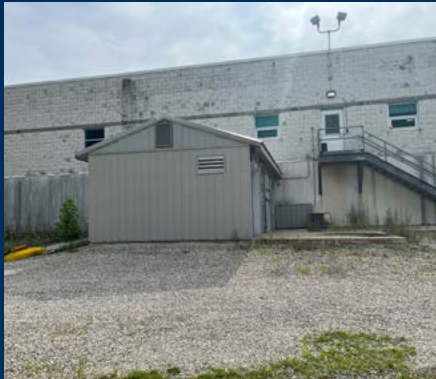
Evaluation will consider improved chlorine storage facilities for better access and staff safety.
